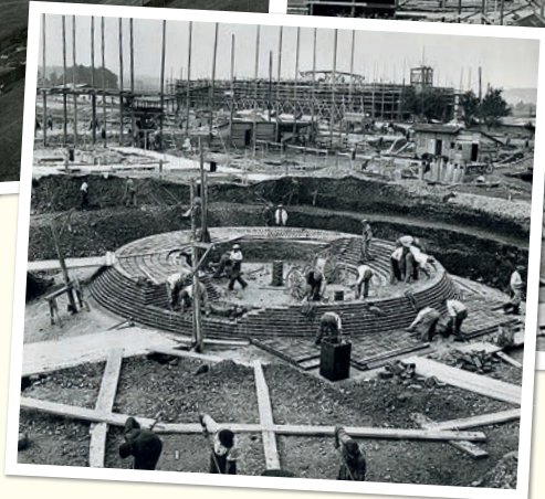
1938 CONSTRUCTION BEGINS ON THE FACTORY—THE SHOKESTACK IS BEING PUTTING UP, AND THE PRODUCTION AND ADMINISTRATION BUILDINGS ARE EMERGING
